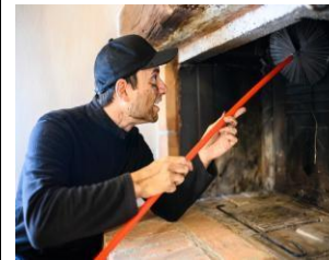
Chimneys and flues
